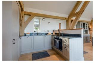
to an exceptional standard. The oak frame was sandblasted to remove marks once the timber/ aluminium composite windows had been installed.
