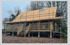
The barn-style home was designed by Roderick James Architects with the oak frame erected in just four days by Post and Beam, a company based in St Ives. The structure was completed with the addition of a standing seam coated-steel roof and structural insulated panels. The oak frame was later sandblasted to remove any marks before being clad in larch.
